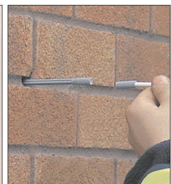
Attach to guider and pull back through
